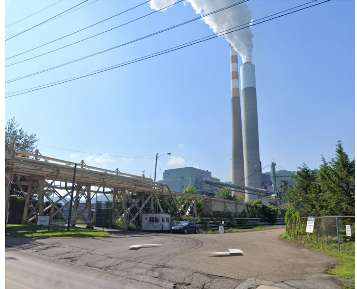
Former powerplant view
